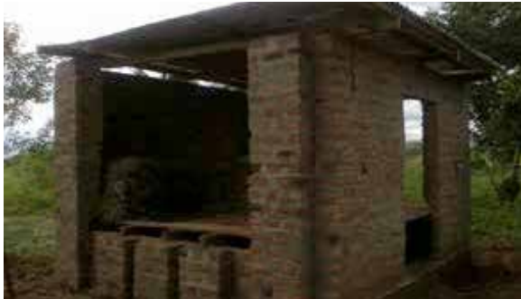
Typical Barns and shelters for Hay storage
