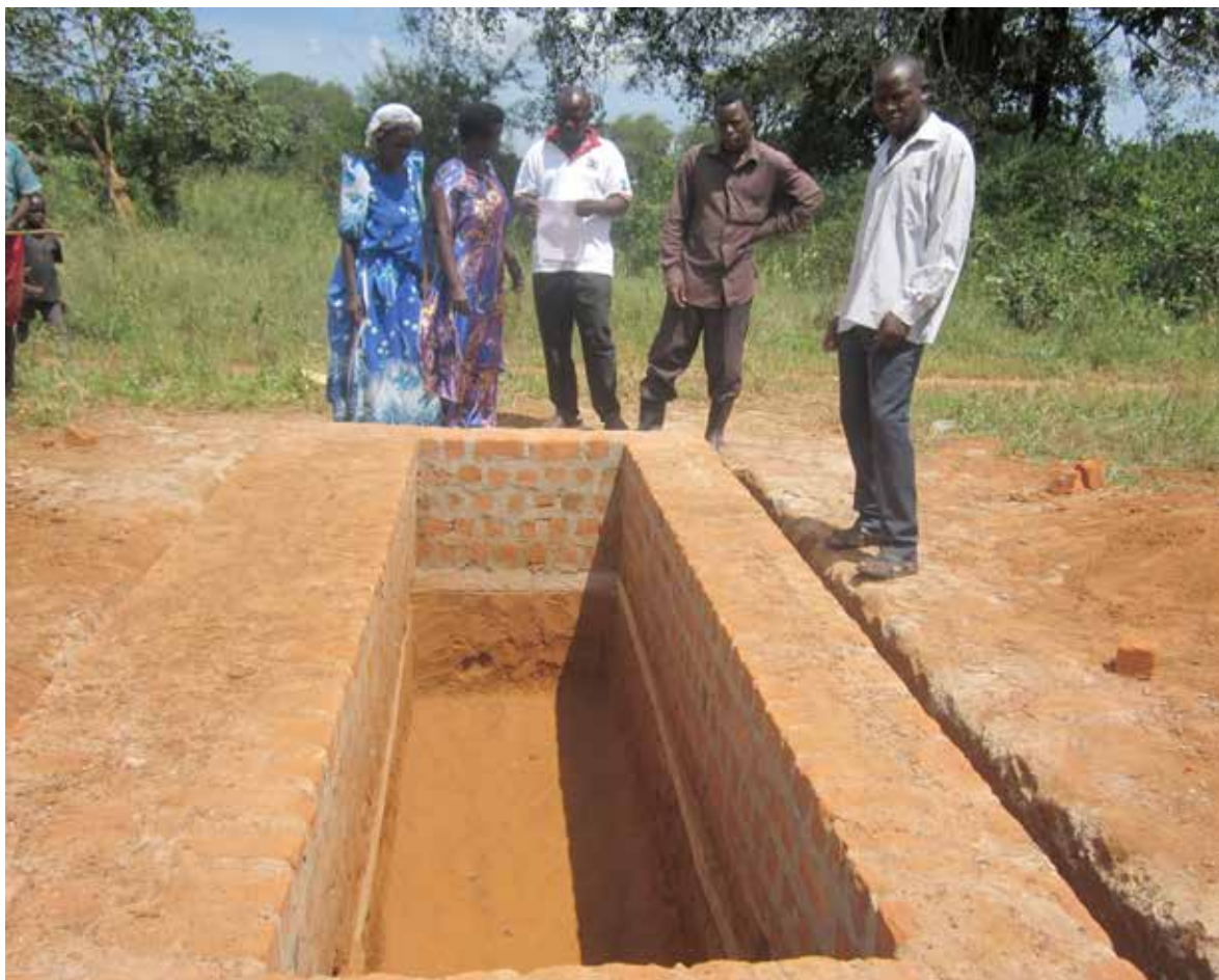
Group members proudly take UNDP staff around a tour of a pit latrine built for TWG
