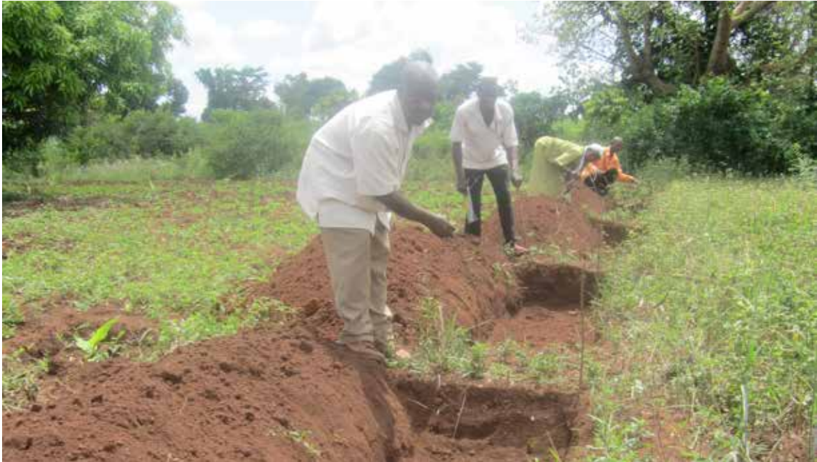
Project beneficiaries construct soil and water conservation structures
