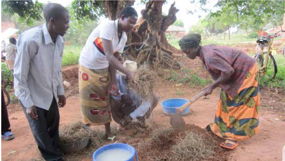
Members prepare the mixture for making stoves
