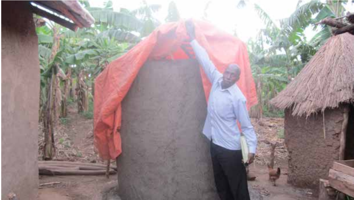
Beijuka shows a member's rain water harvesting tank under construction.
