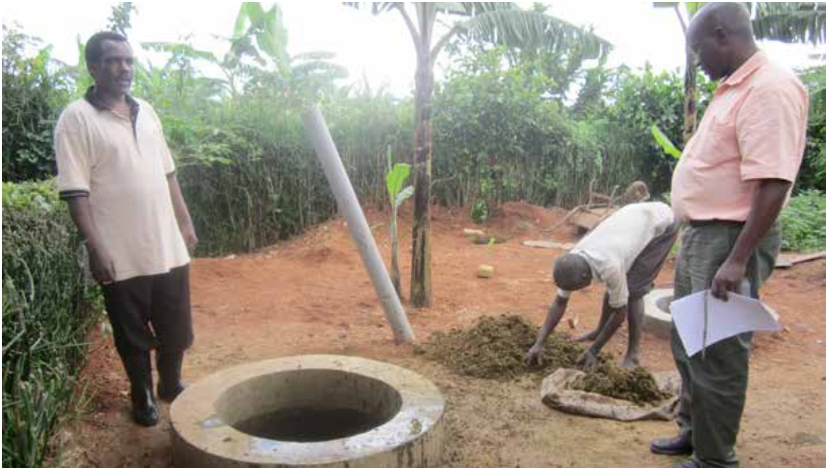
Asiimwe supervises the feeding of his Bio-gas digester
